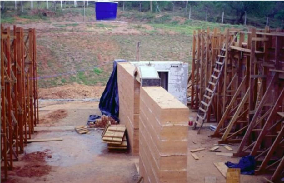
img. 6 - Images of the construction site of the Gilda Barros house, in which we observe mud walls, stone foundations and strategies used on the roof (Photos: Fernando Minto, involved in the construction).
